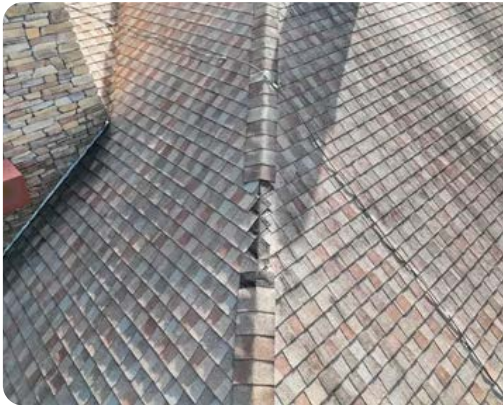
Another section of damaged hip & ridge shingles.
