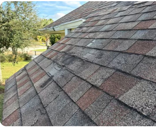
Another view of damaged shingles.
